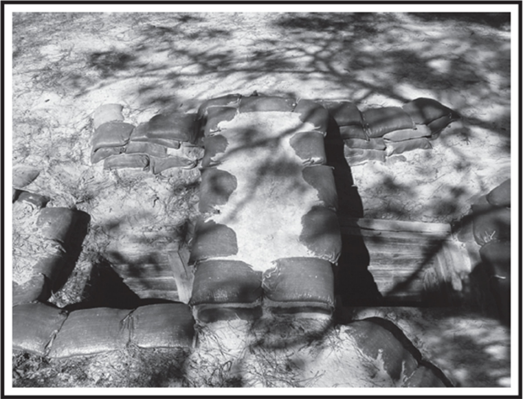
071-COM-4408-8. Machine gun fighting position with OHC.
