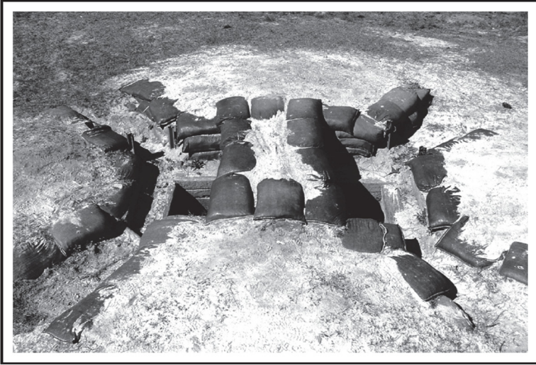
Figure 071-COM-4408-2. Two-man fighting position with OHC.
